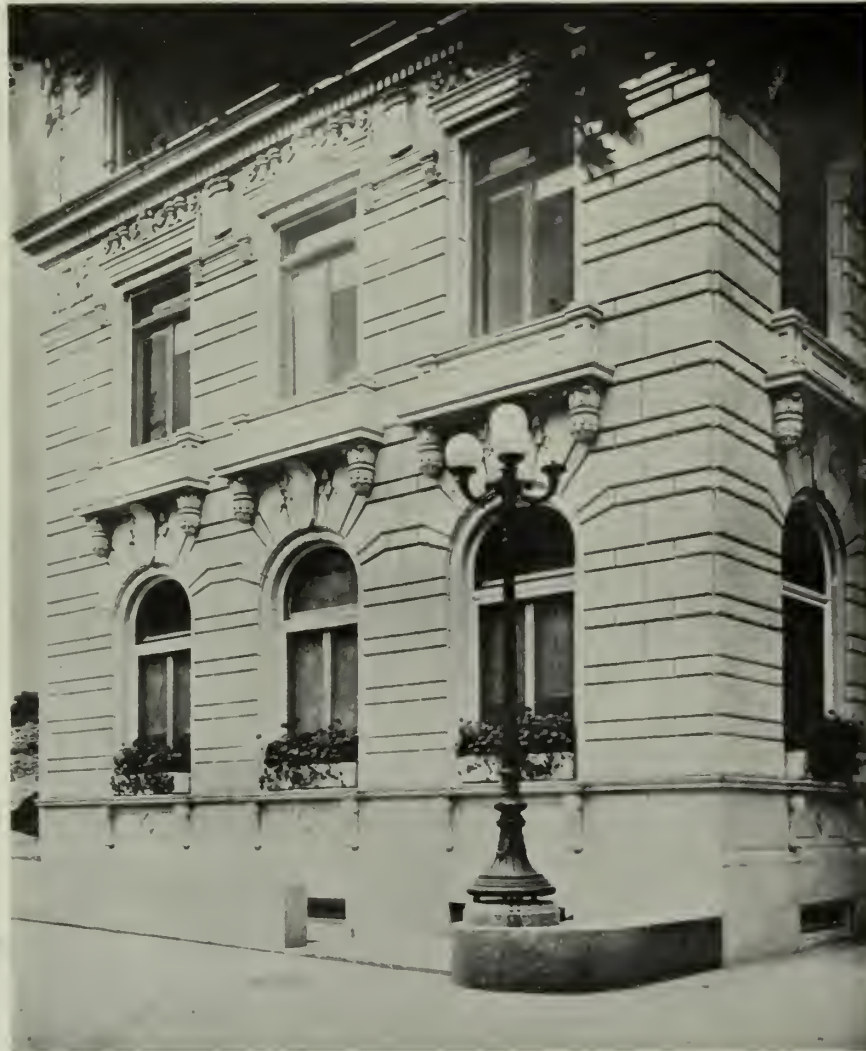
DETAIL OF APARTMENT HOUSE, RIVERSIDE DRIVE, NEW YORK CITY. Executed in white mat terra cotta by New York Architectural Terra Cotta Company. G. Ajello, Architect.
